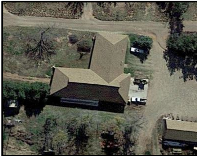
Tucumcari Shop and Storage roof view
