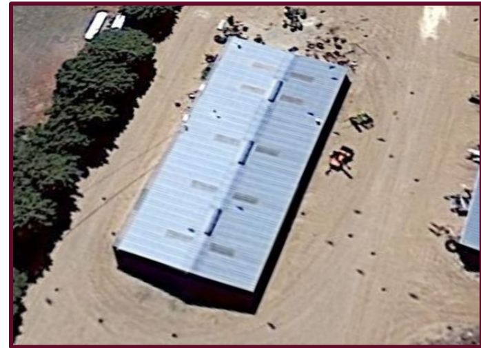
Farmington Shop roof view
