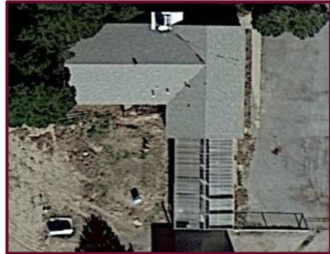
Artesia Office-roof view
