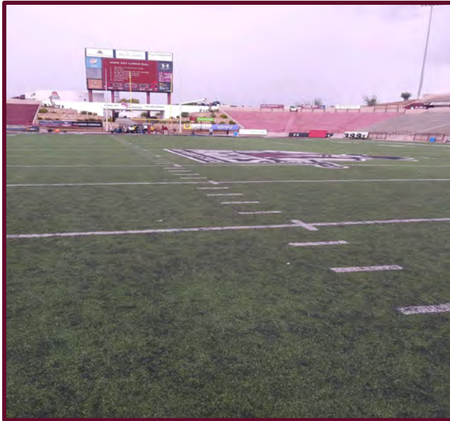
Aggie Memorial Stadium playing field with rubber mat exposed due to wear
