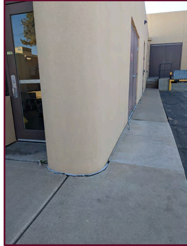
Foundation settlement at building on east and north sides of building #330
