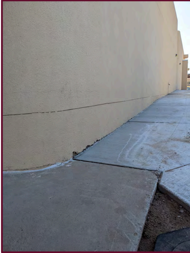
Foundation settlement at building on east and north sides of building #330
