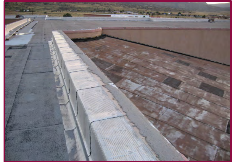
Martinez Hall main entrance view from the top showing roof parapet deterioration and aging roof in need of replacement
