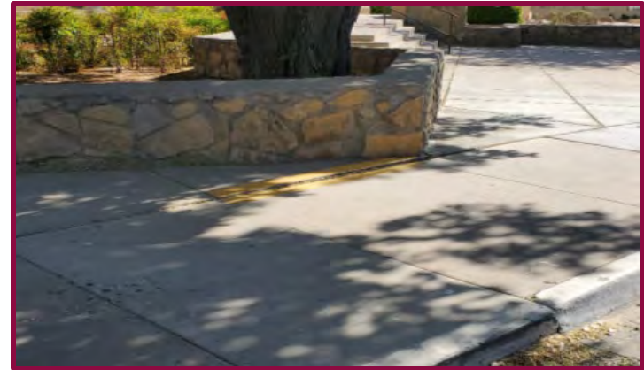
Remove and replace existing broken concrete trip hazards
