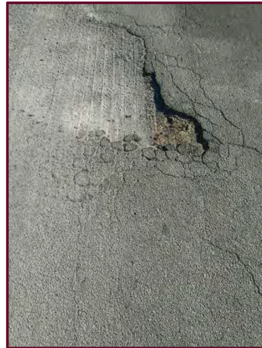
Visible distress showing block cracking and severe surface raveling
