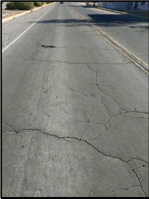
Visible distress showing longitudinal and transverse cracks
