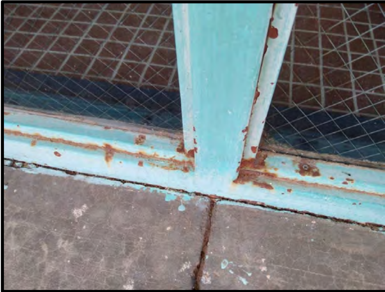
Exterior window & frame
