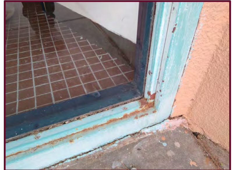
Exterior window & frame
