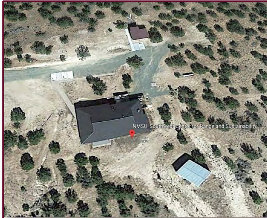
Aerial View of the site
