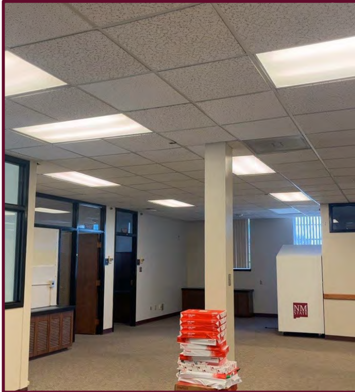
Office Suite suspended ceiling system
