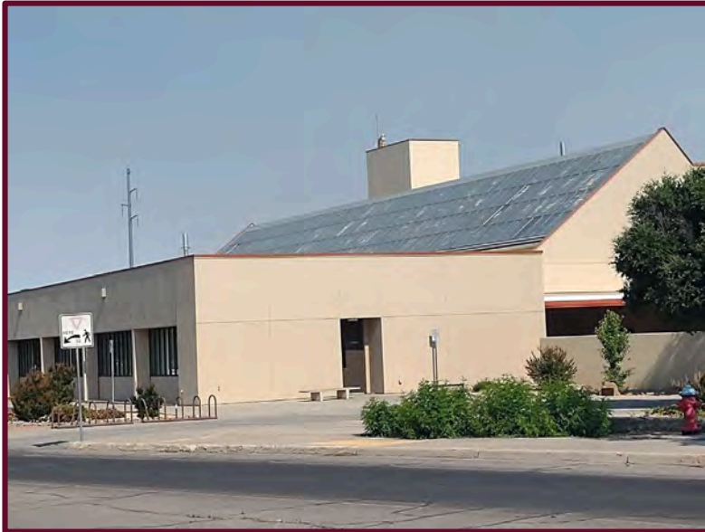
Engineering Complex I (ECI) looking northwest
