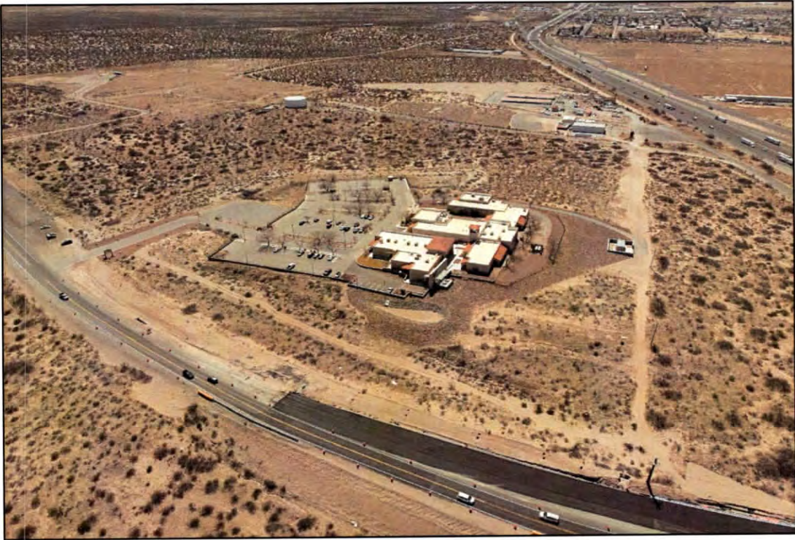
View looking south across the subject from above NMSR 404.
