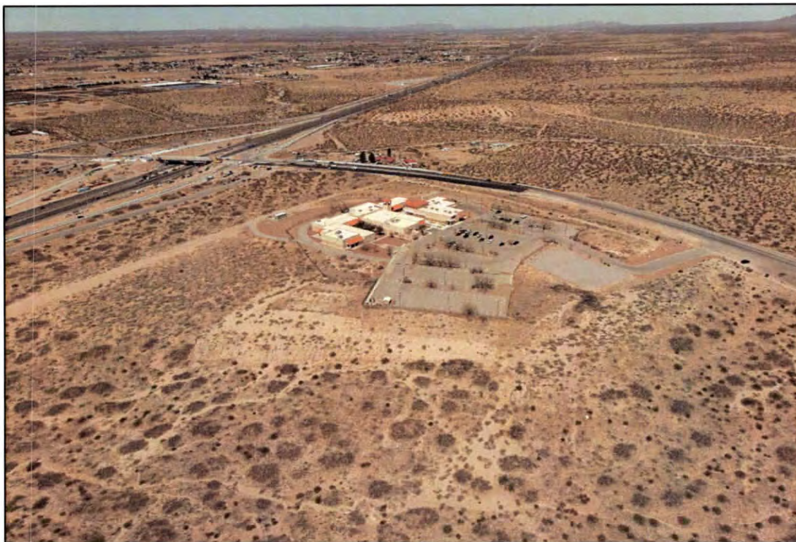
View looking north across the subject from above the southwest property corner.
