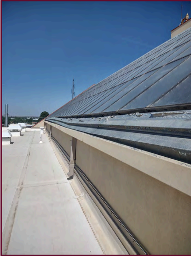
Engineering Complex I (ECI) images of existing solar panels
