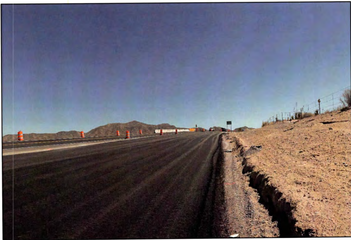
View looking east along NMSR 404. Subject is on the right.
