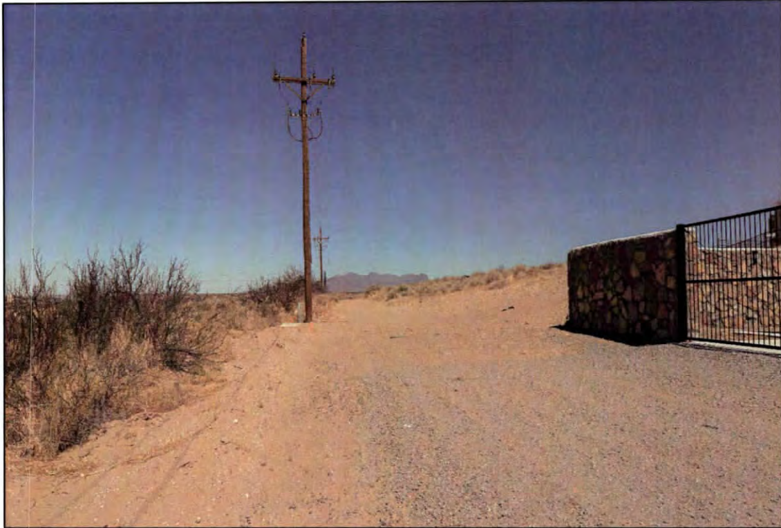
View looking north along the subject's west property boundary. The newly constructed utility structure is on the right.
