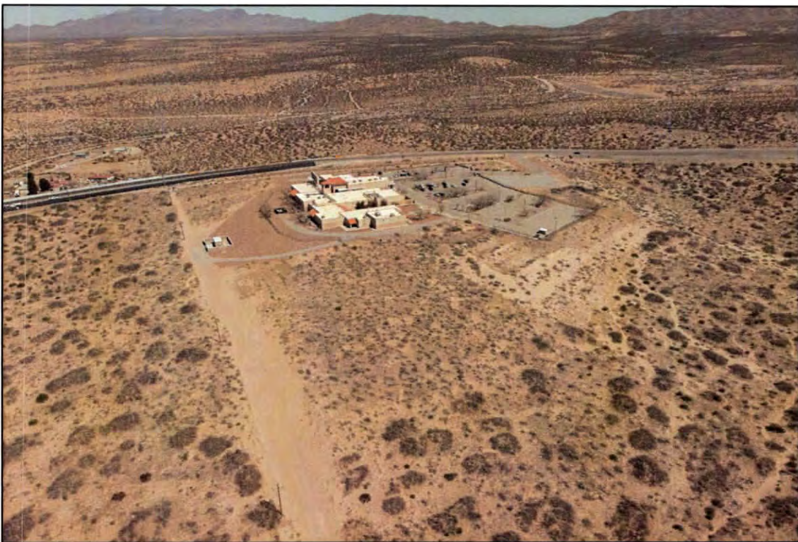
View looking north along the subject's east property boundary.
