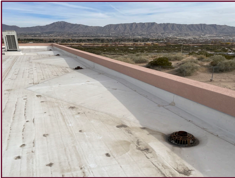
DACC Sunland Park Center-Roof
