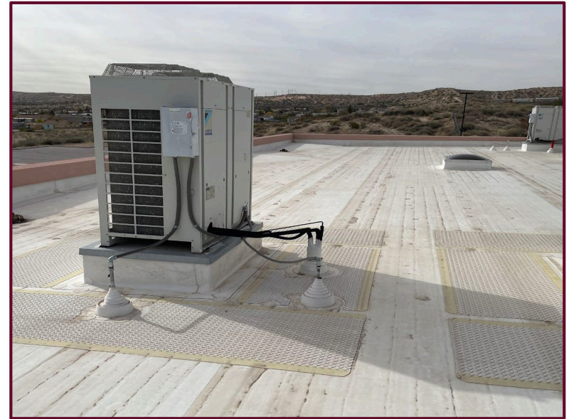
DACC Sunland Park Center-Roof
