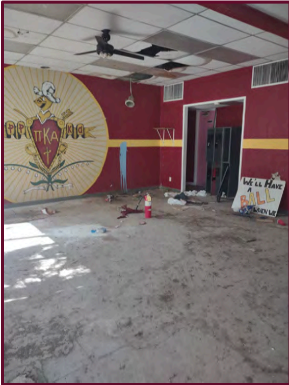
Greek East interior images of lounge area and water damage ceiling
