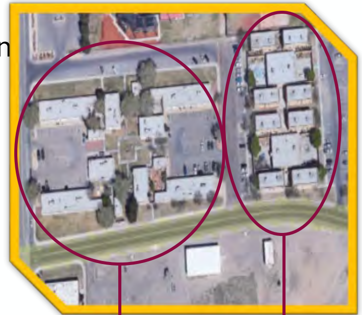
Greek West (Building # 271 to 274)
