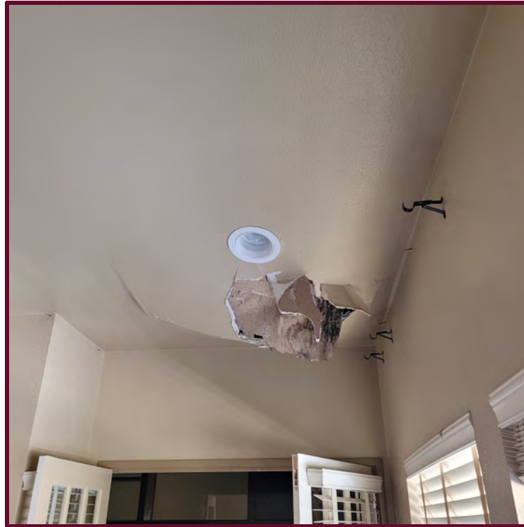
Greek East interior images of lounge area and water damage ceiling
