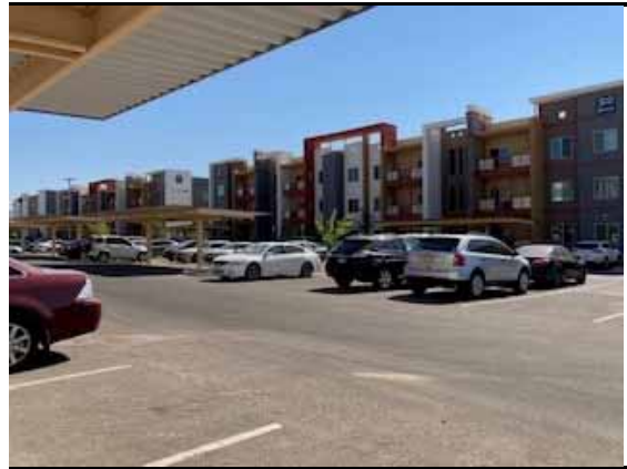
View of the typical apartment building façade.
